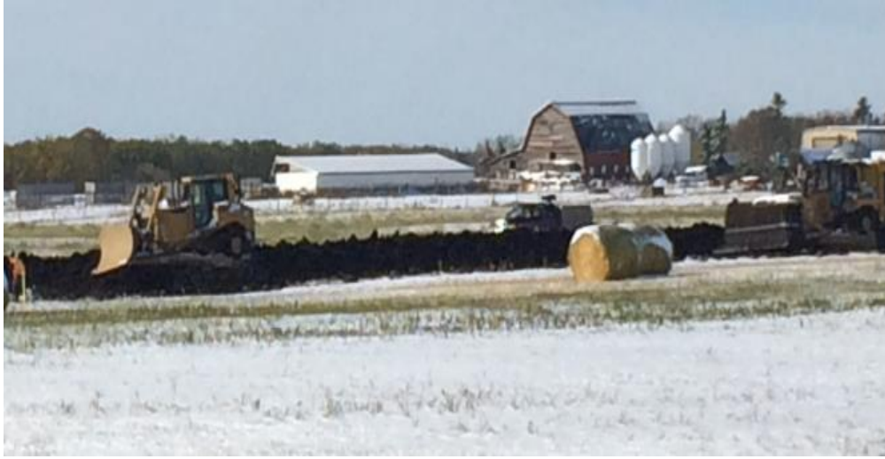
Power dozer stripping topsoil 707 + 757
